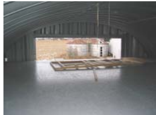
The view to the outside from the second floor of quonset hut #2.
