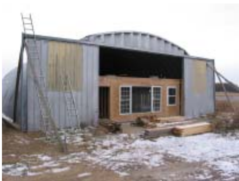
View of quonset hut #2 with new doorway and windows.
