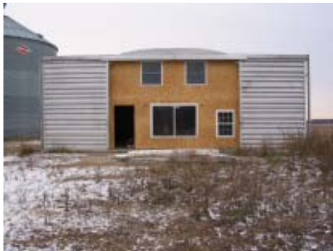
Front view of quonset hut #1 with newly installed windows and doorway.
